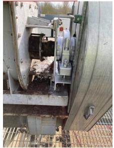
EMERGENCY complex repair and modifications to replace both bearings on Cake Silo Auger. Customer very pleased as there was no down time in production and the site continued to run as normal. This also improved the future maintenance of the bearings.
